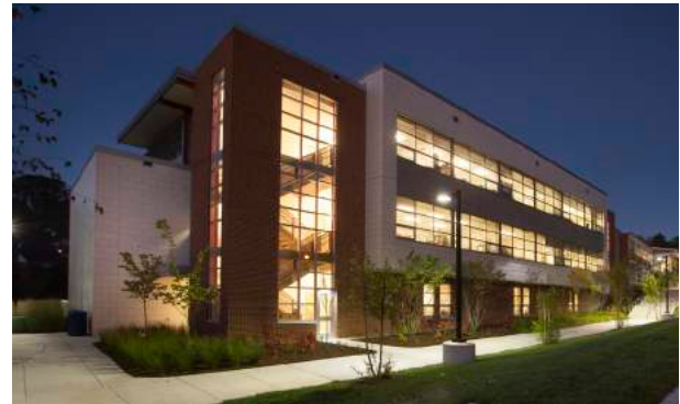
Grunley used BIM to model systems and prevent clashes during the Ashlawn Elementary School Renovation and Addition project in Arlington, VA (shown above). BIM allowed us to complete the installation of new systems within the addition, upgrade systems in the existing building and tie-in new systems to the existing systems while the school remained operational without disrupting daily activities.
