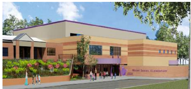
Grunley and are currently providing design and construction services for renovations and additions to the Mount Daniel Elementary School for the City of Falls Church under a PPEA contract.
