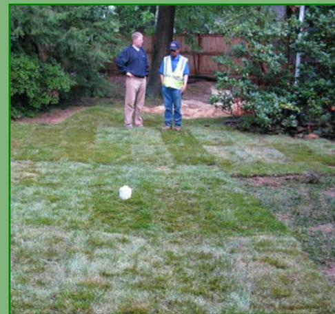
Once installed, the infiltration trench is invisible except for a short portion of PVC pipe used to maintain the trench.
